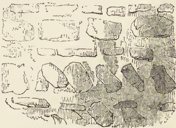
19. Rubble Masonry, Gundulph's Tower, called St. Leonard's, at Malling, Kent, A.D. 1070.
